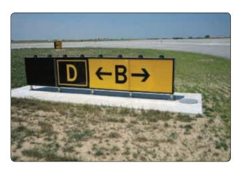
**Figure 14-18.** Taxiway Bravo direction sign with a collocated Taxiway Delta location sign. When the arrow on the direction sign indicates a turn, the sign is located prior to the intersection.
