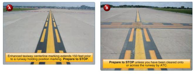
Figure 14-21. (A) Enhanced taxiway centerline marking. (B) Enhanced taxiway centerline marking and runway holding position marking.
