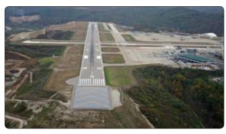
Figure 14-55. Engineered material arresting system (EMAS) located at Yeager Airport, Charleston, West Virginia.
