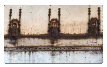
Figure 8-18. Galvanic corrosion.
